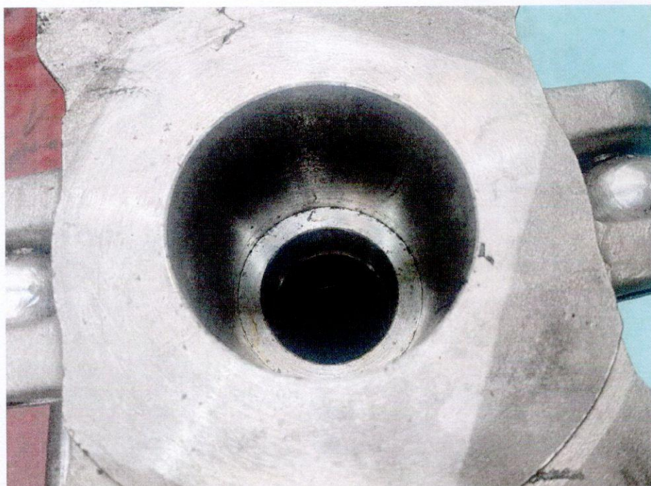
填料函 Packing sealing chamber
