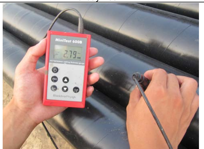
Coating layer thickness check
