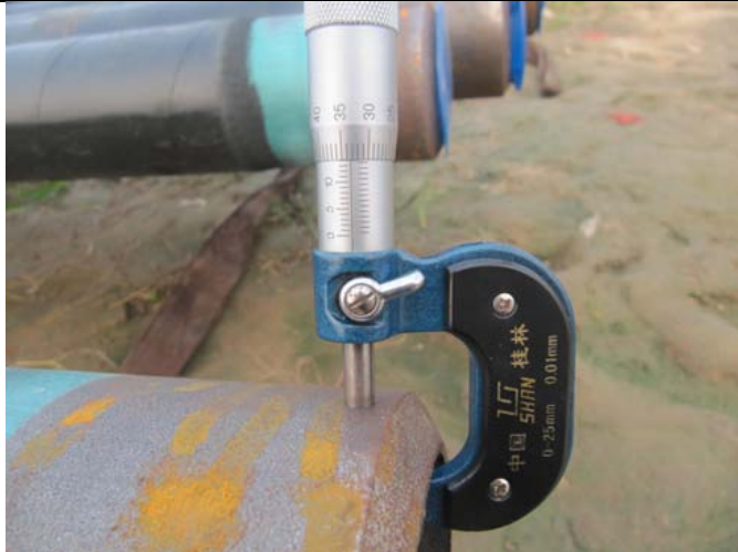
Pipe wall thickness check
