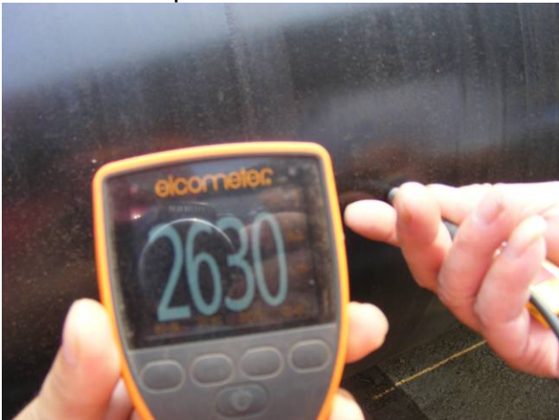
Total thickness of 3PE coating check
